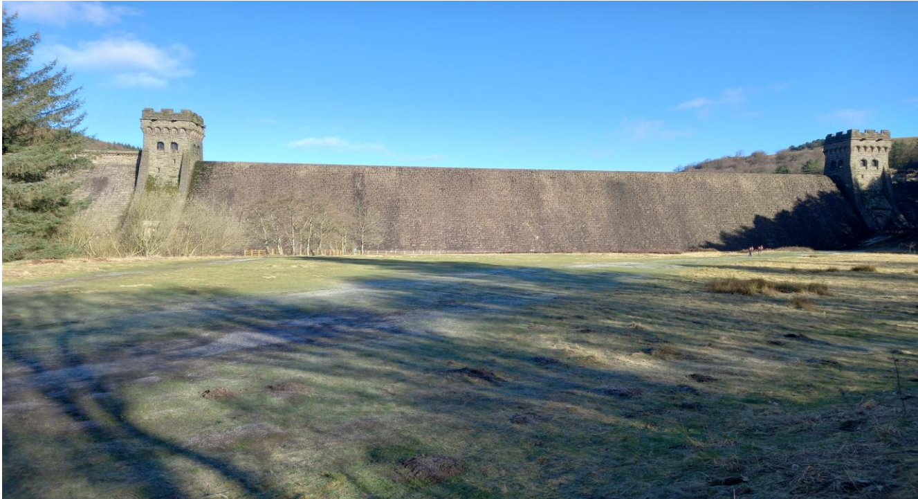
Derwent Dam wall showing the 2 towers
