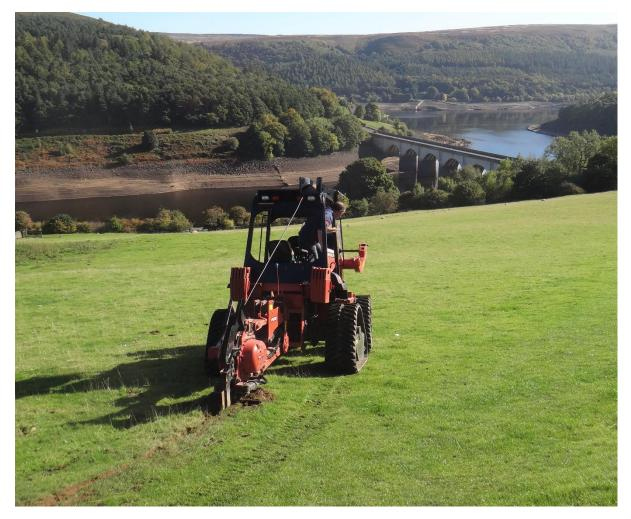
The 'Ditch Witch' vibrating mole plough (M Downes Earthworks Ltd) burying the new cable.
