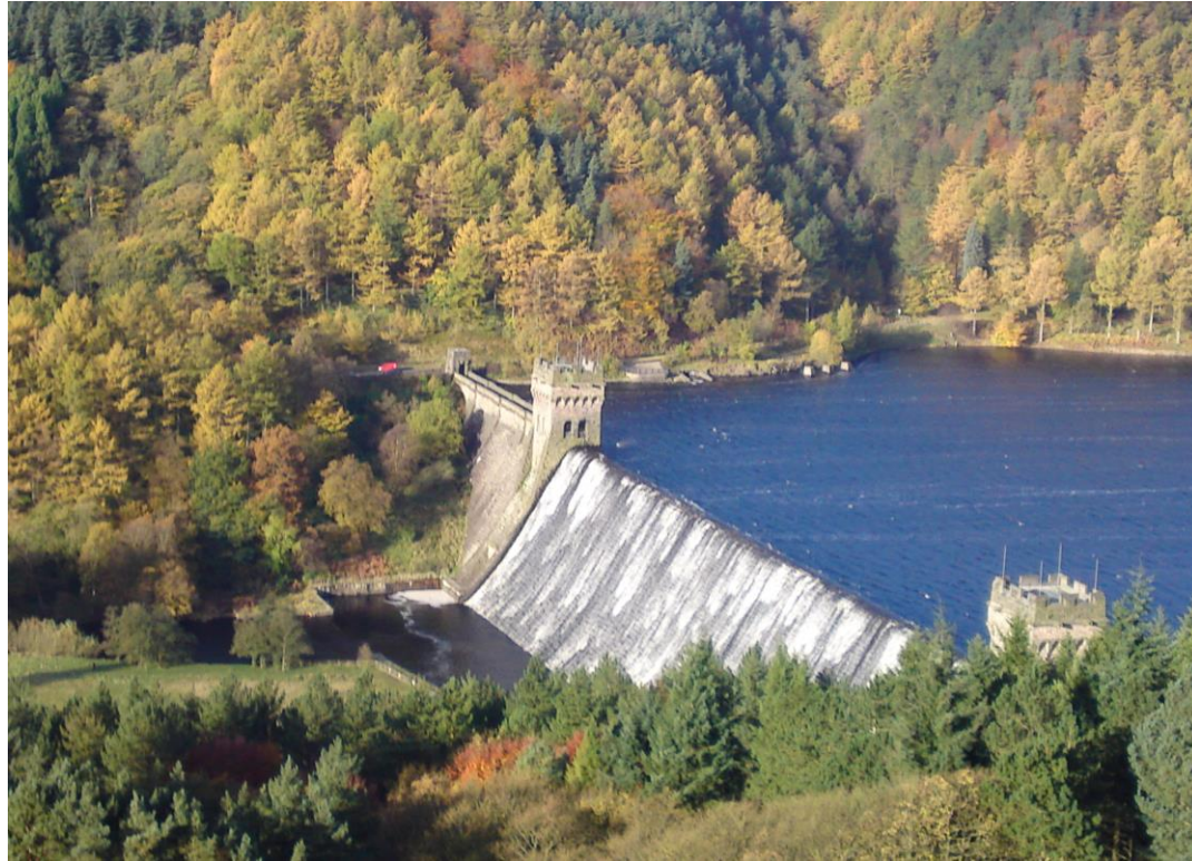
Derwent Dam wall
